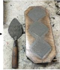
Leveling the mortar
