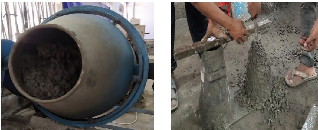
Figure 6.11: Mixing of Concrete
