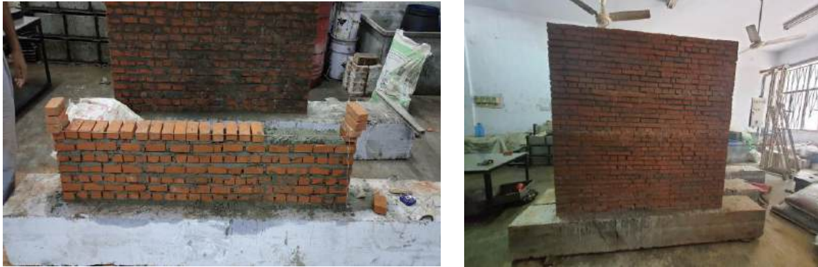
Figure 3.22- URM wall construction
