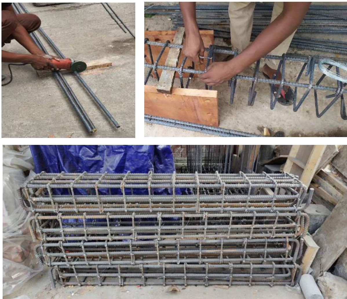
Figure 3.13- Reinforcement Preparation for base of RM walls.
