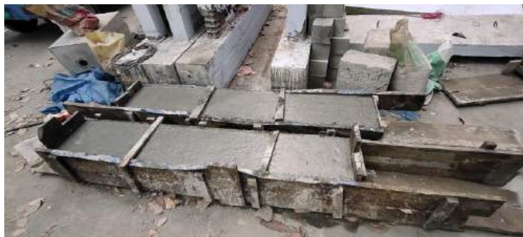
Figure 3.21- Base Construction for URM.
