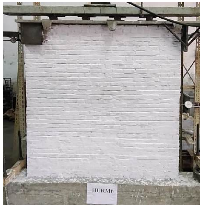
Figure 3.23- URM wall after whitewash.
