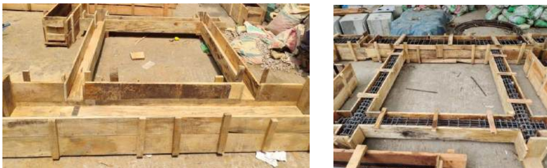
Figure 3.25- Shuttering work.
