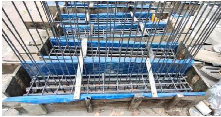
Figure 3.15- Formwork Preparation of RM walls
