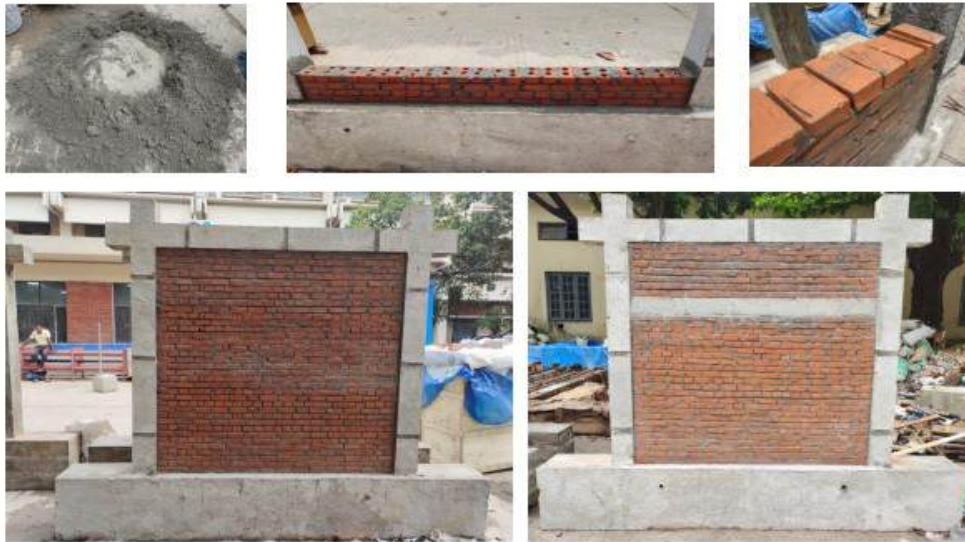
Figure 3.28- Masonry work for Infilled Frame.
